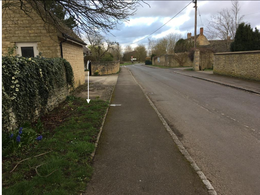
Location 8 Church Road outside Blacksmiths Close
